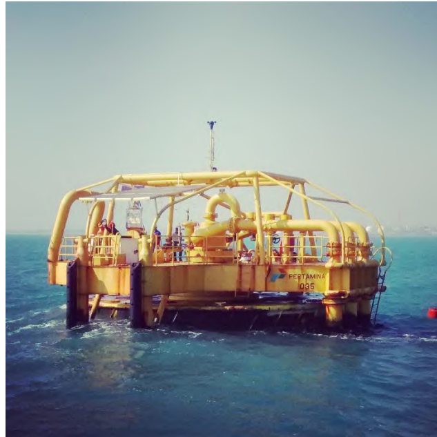
Gambar 4.1. SPM ( Single Point Mooring ) 035 Pertamina TBBM Tuban (Sumber : Dokumen Pribadi)
