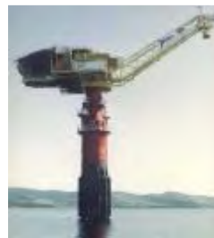
Gambar 2.4. Articulated loading platform (ALP) (Stella, 2012)
