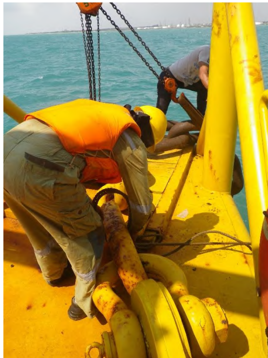
Gambar 4.16. End Joining Shackles (Dokumentasi Pribadi)
