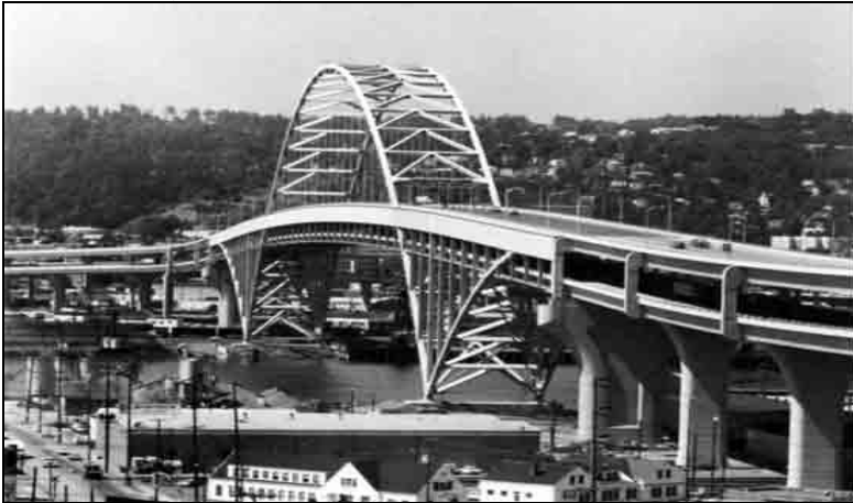
Gambar 2.3 Jembatan tipe A half – Through Arch
