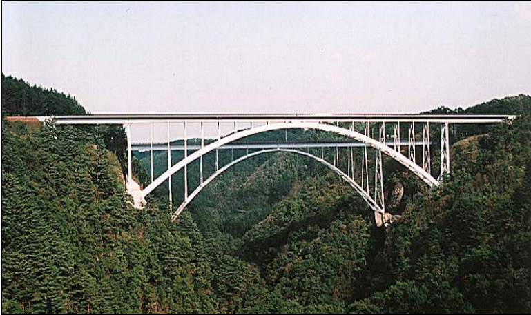
Gambar 2.1 Jembatan tipe Deck Arch
