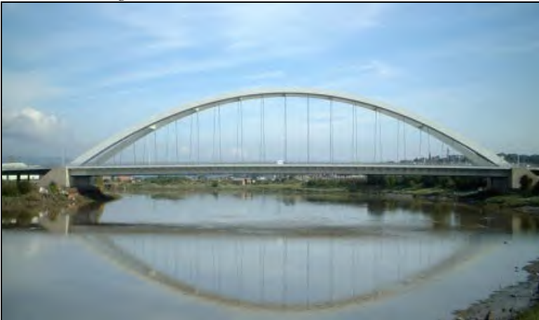
Gambar 2.2 Jembatan tipe Through Arch
