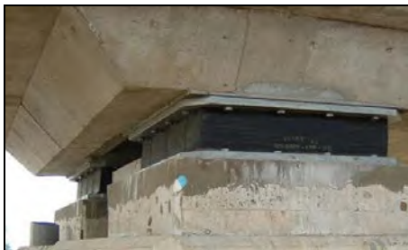
Gambar 2.19 Perletakan Elastomer Bearing
