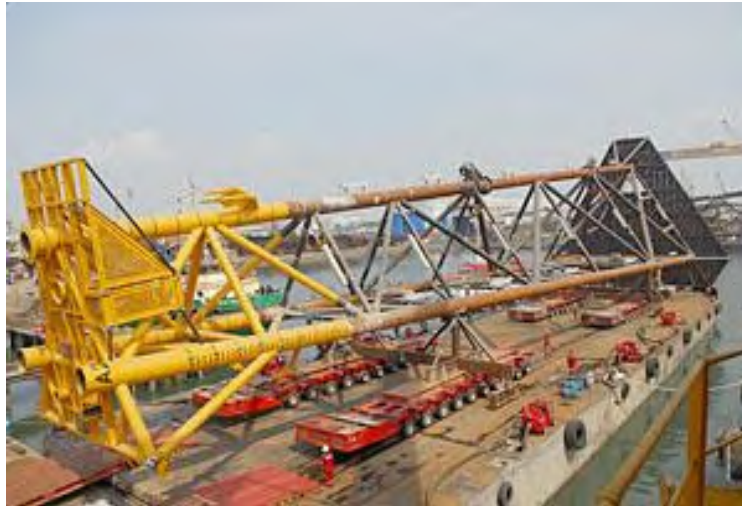
Gambar 2.5 Fabrikasi Well Head Sumur migas Santos (Madura Offshore)
