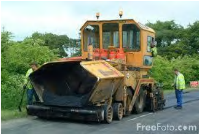
Gambar 5.9. Peralatan Aspal Finisher
