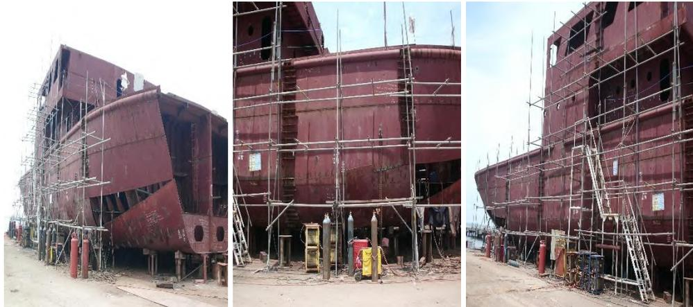
Gambar 4.19. Proses *erection* kapal perintis 750 DWT di PT. ASSI
