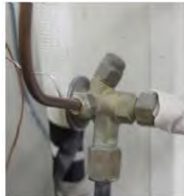
Gambar 3.8 Valve TXV
