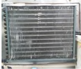
Gambar 3.4 Kondensor High stage
