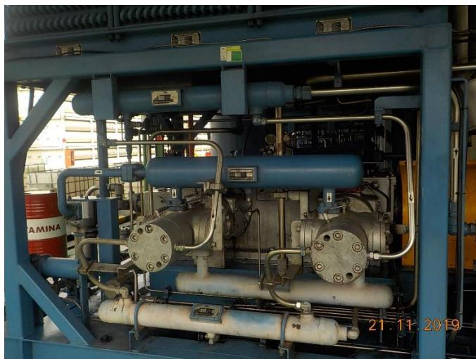
**Gambar 2.4 Kwangshin CNG Compressor**
