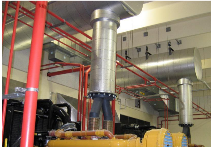
Gambar 2.9. Gambar Silencer gas buang
