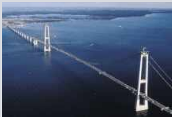
Storebælt East Bridge, Denmark built: 1996 Suspension bridge main span: 1624 m type of joint: DS2000 51.40 lin. metres DS1520 25.70 lin. metres DS1200 25.70 lin. metres DS960 25.70 lin. metres DS800 25.70 lin. metres
