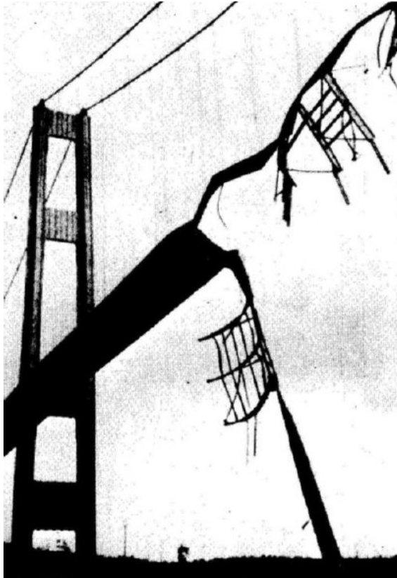
Gambar 2. 32 Keruntuhan Jembatan Tacoma Sumber : (E-book Cable Supported Bridges, Niels J. Gimsing, 2012)
