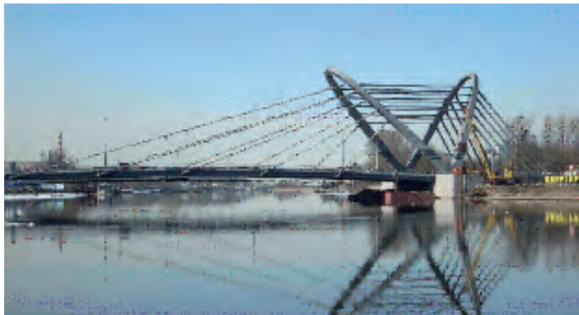
Lazarevskiy bridge, Saint Petersburg, Russia (2008) Stays ranging from 6-55 to 6-73
