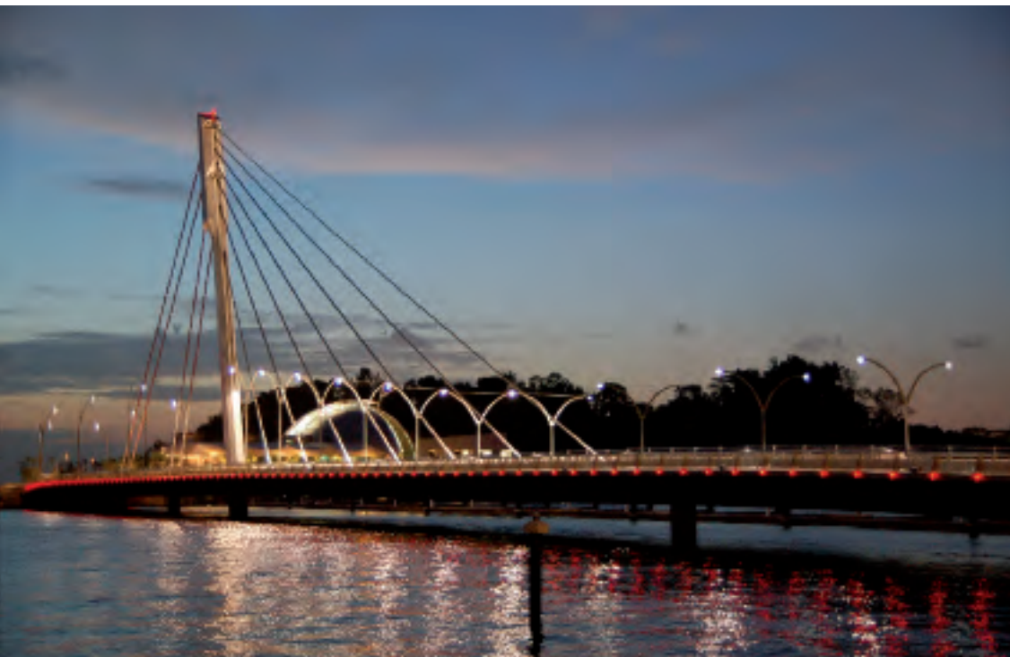
Keppel Bay Bridge, Singapore (2006) Supply and operation of fastening cells, erection of bridge deck, pylon construction, supply and installation of stay cables
