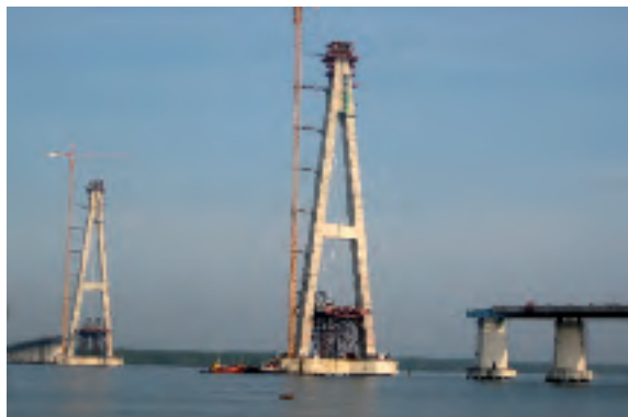
Sungai Johor Bridge, Malaysia (2008) 85 strand cables with length up to 275m
