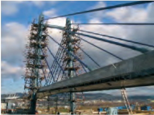
Zizkova Footbridge, Czech Republic (2007) Installation of stays and post-tensioning
