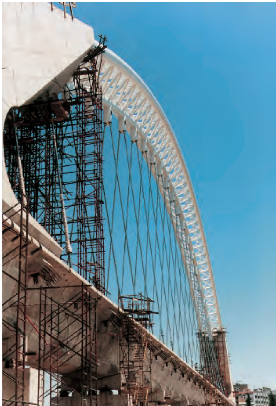
Merida Arch Bridge, Spain (1991) Supply and installation of the stay cables
