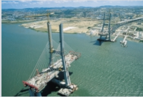
Vasco da Gama Bridge, Portugal with fuse box for earthquake movements built: 1997 Cable-stayed bridge main span: 829 m type of joint: DS1440 59.00 lin. metres
