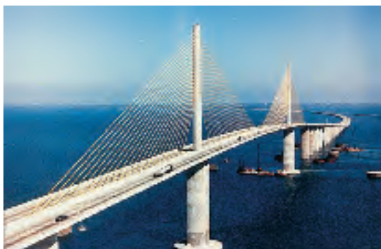
Sunshine Skyway Bridge, USA (1986) Supply of post-tensioning and stay cables. Cables anchored to the pylon by saddles and equipped with hydraulic dampers
