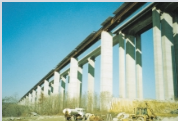
Stura di Demonte, Italy built: 1999 Composite steel bridge length of bridge: 2750 m type of joint: DS1200 24.50 lin. metres
