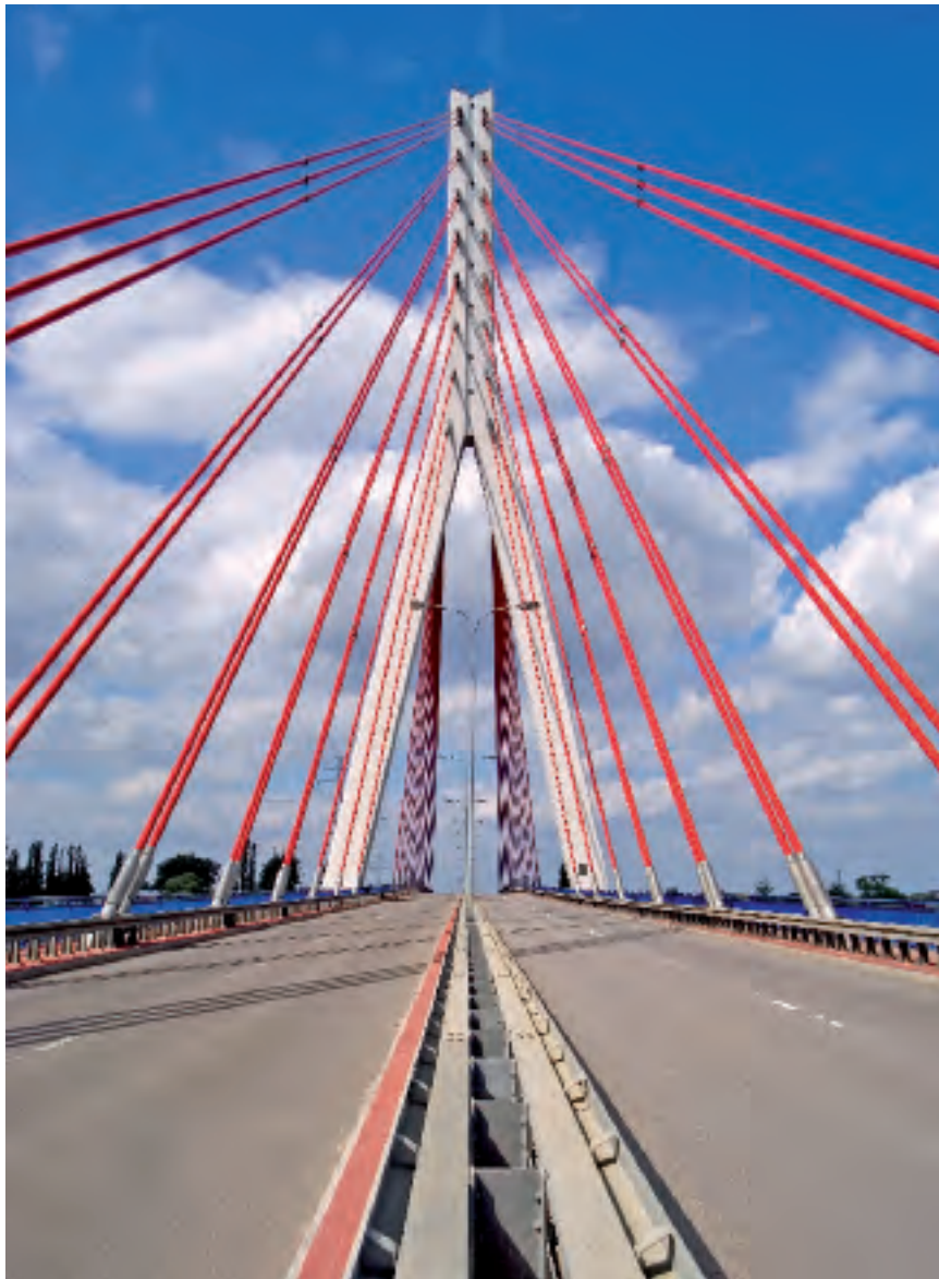
Sucharskiego Bridge, Poland (2001) Supply and installation of stay cables, with VSL Friction Dampers
