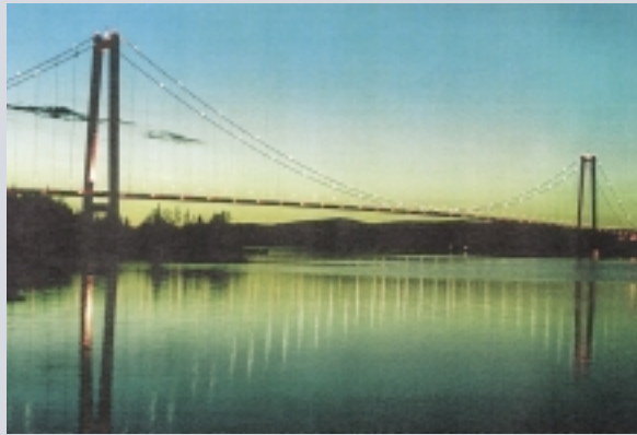
Höga Kusten Bridge, Sweden built: 1997 suspension bridge main span: 1210 m type of joint: DS1840 36.80 lin. metres
