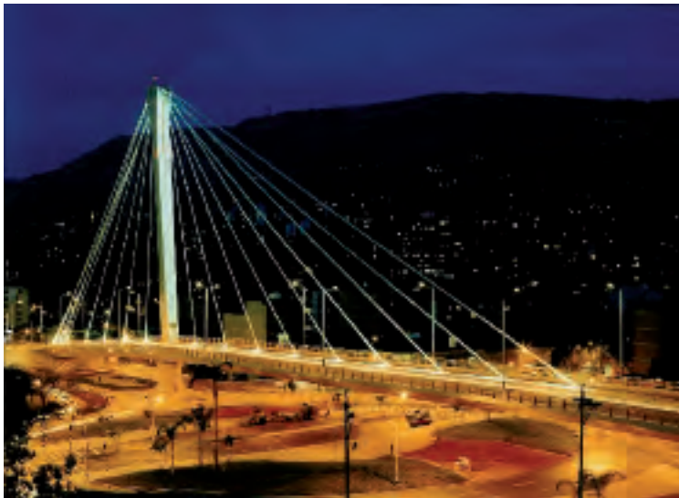
Peldar Bridge, Columbia (2002) VSL Saddle and monitoring services
