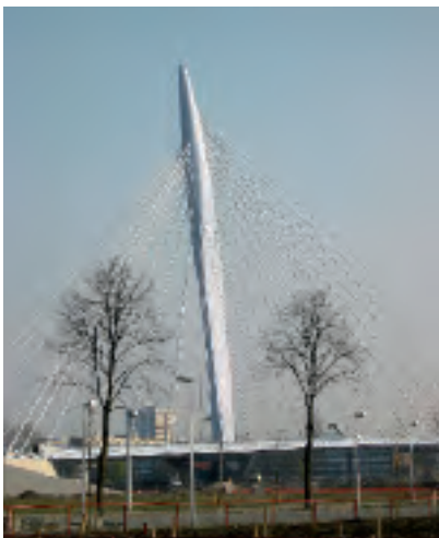
Papendorpse Bridge, Netherlands (2002) 120 strand cables
