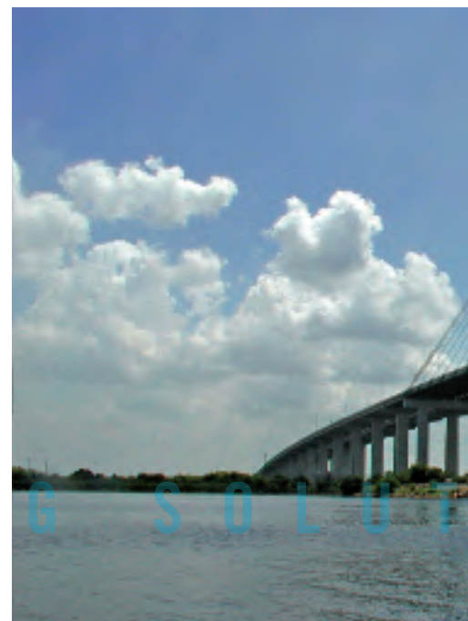
Fred Hartmann Bridge, USA (1995) Supply of stay cables and supervision at installation
