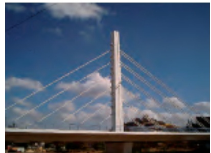
Liz Bridge, Portugal (2004) 18 stay cables installed in one week
