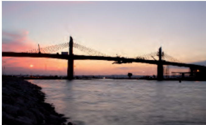
Rades-la-Goulette Bridge, Tunisia (2007) Extensive equipment and services
