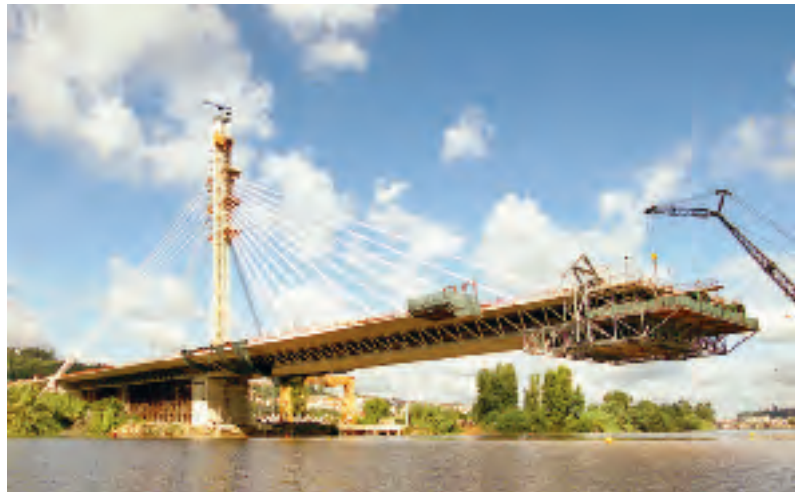
Ponte Europa Bridge, Portugal (2002) 186m main span length - 91 strand cables
