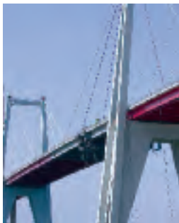
Figueira Da Foz Bridge repair - Portugal
