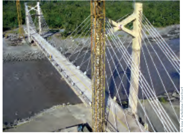
Pastaza Bridge, Ecuador (2005) Supply and installation of the stay cables
