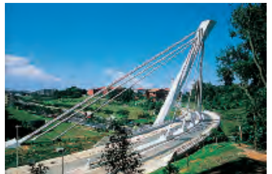
Safti Bridge, Singapore (1995) An inclined pylon is stabilised by back-stay cables
