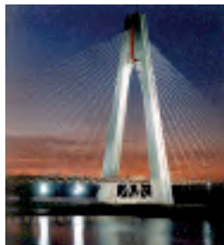
Badajoz Bridge, Spain (1994) Cables equipped with friction dampers
