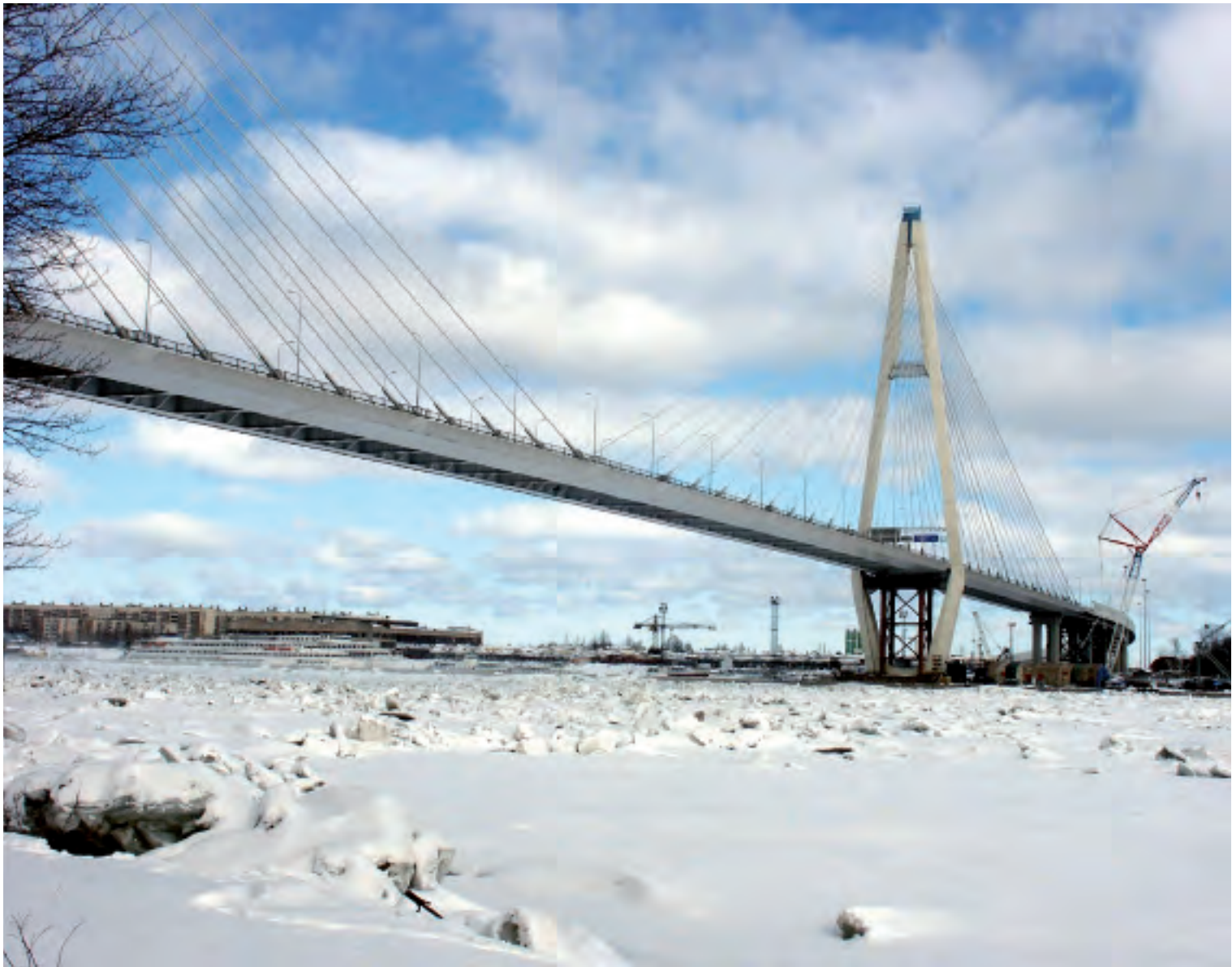
Neva 1 Bridge, Russia (2002) All cables equipped with VSL Friction Dampers
