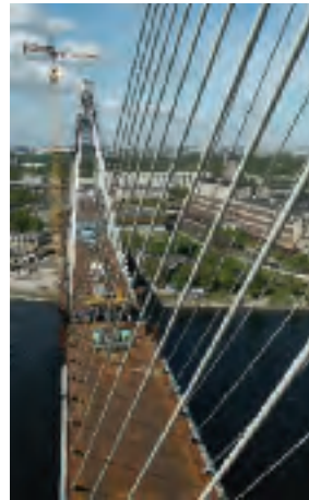
White color stay pipes (Neva Bridge, Russia)
