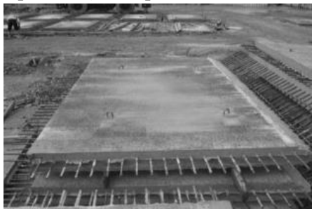
Gambar 4.1 Ilustrasi Half Slab Precast (Irawan, 2017)
