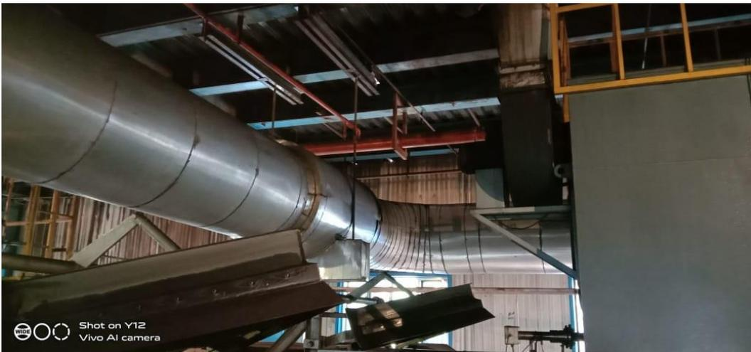
**Gambar 4. 14** Pipa *line steam* di area BC 6
