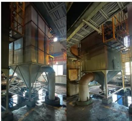
**Gambar 4.13 Dust Collector Area Tripper PLTU Pacitan**
