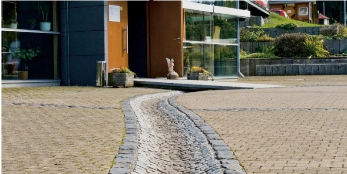
Figure 15. An example of an above ground drainage in the street. (Urban Green-Blue Grids, 2020)
