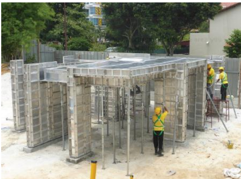
Gambar 4.44 Aluminium Formwork System
