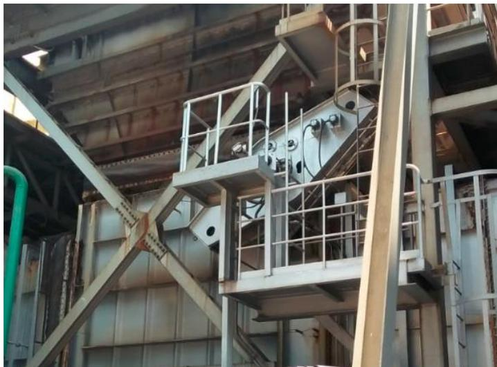
Gambar 2.8 *Expantion Joint*
