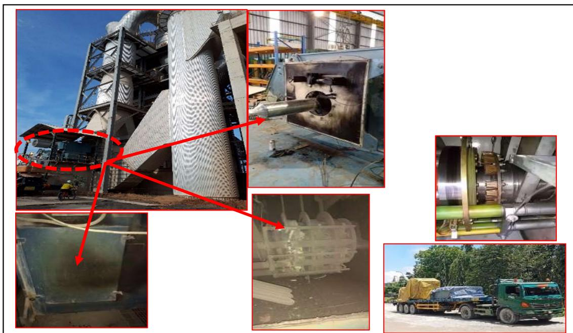
Gambar 1.5 *Problem di area Motor Fan 341FN2 Raw Mill 7100 kW, Spare Parts Electrical Brush Lifting Device (BLD) Mengalami Stockout*
