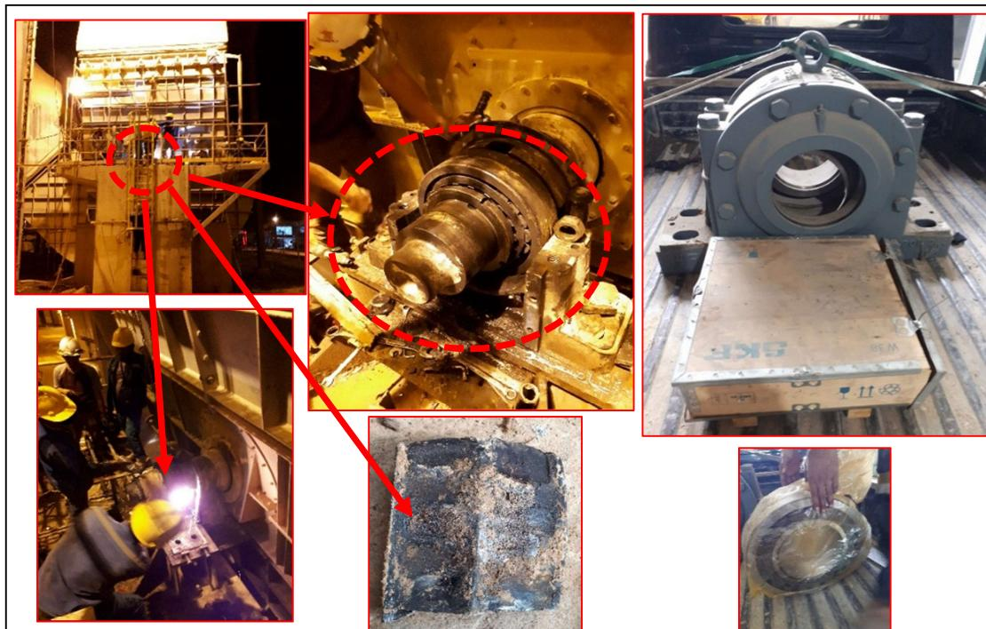
Gambar 1.4 Problem di Area Fan Main Bag Filter 341FN3 Raw Mill, Spare Parts Bearing Mengalami Stockout
