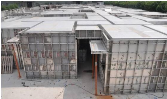
Gambar Aluminium Formwork (Sumber : Prasanth S)
