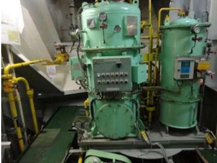
Gambar 2. 5 Oily Water Separator
