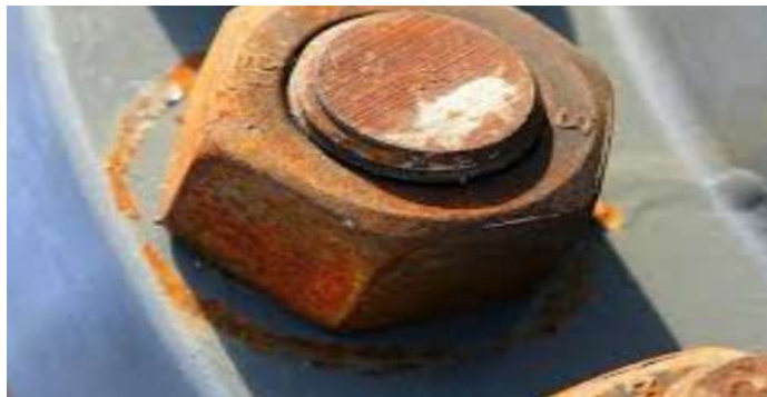
Gambar 2.8 Contoh tipe Galvanic Corrosion
