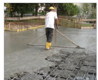
Photographic details of the complete sequence of positioning the scaffolding, positioning the U-Boot Beton ® , reinforcement of the structure to be performed on site, casting and final smoothing.
