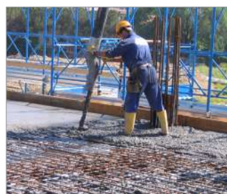
Photographic details of the complete sequence of positioning the scaffolding, positioning the U-Boot Beton ® , reinforcement of the structure to be performed on site, casting and final smoothing.
