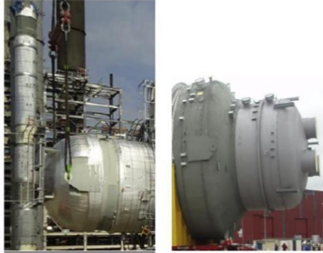
Gambar 2.6. Side mounted top lug (sumber: Antalfy dkk, 2016)
