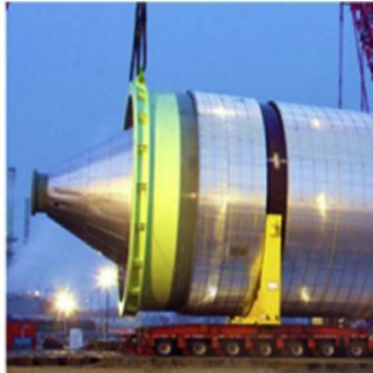
Gambar 2.8. Skirt tailing lug (sumber: Antalffy dkk, 2016)
