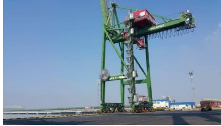
Figure 2.3 Ship To Shore Container Konecranes
