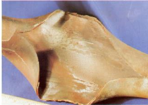
Gambar 2. 13 Violent Ruptured pada Super Heater akibat Short Term Overheating (Port, Herro and Robert, 1991)
