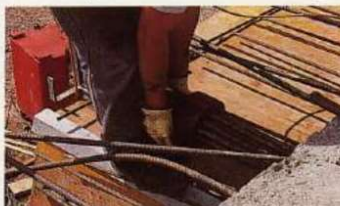
Placing of anchor head
