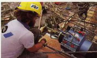
Stressing, measuring, seating of wedges
