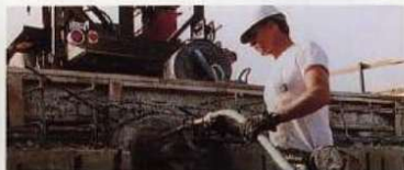
Grouting of tendon
