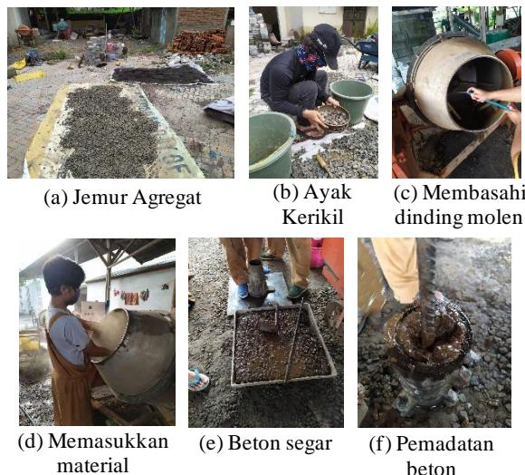
Gambar 3.7 Pengecoran Beton Geopolimer
