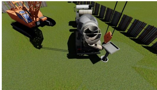
Gambar 5.52 Pengecoran Ready Mix kedalam Bored Pile
