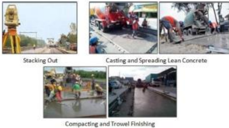
Gambar 4. 17 Pekerjaan Lean Concrete
