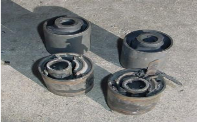
Gambar 2.15 Kerusakan Steel Rubber Bushing
