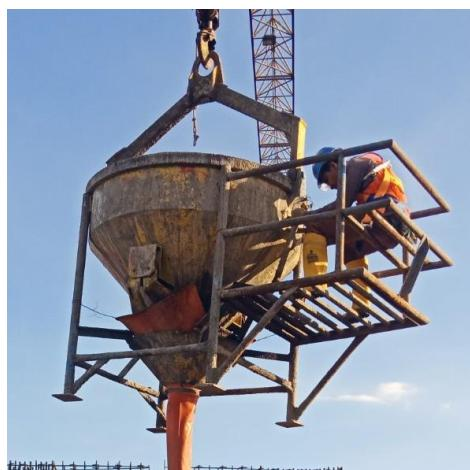
**Gambar 2.8 Concrete Bucket**
