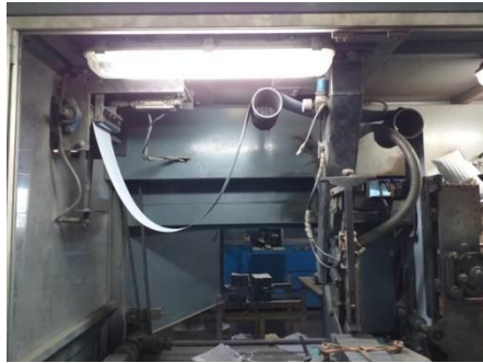
Gambar 2. 5 Separator Transport System
