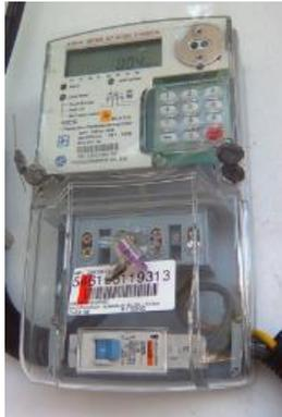
**Gambar 2.2.** KWH Meter Digital
