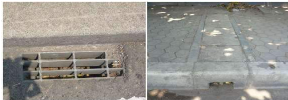
(a) Inlet got tepimendatar (b) Inlet kerb tepi
