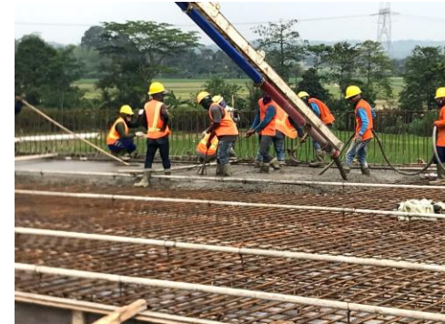
Pengecoran deck slab
