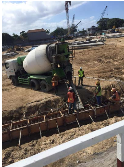
Gambar 4.10 Pengecoran Capping Beam
