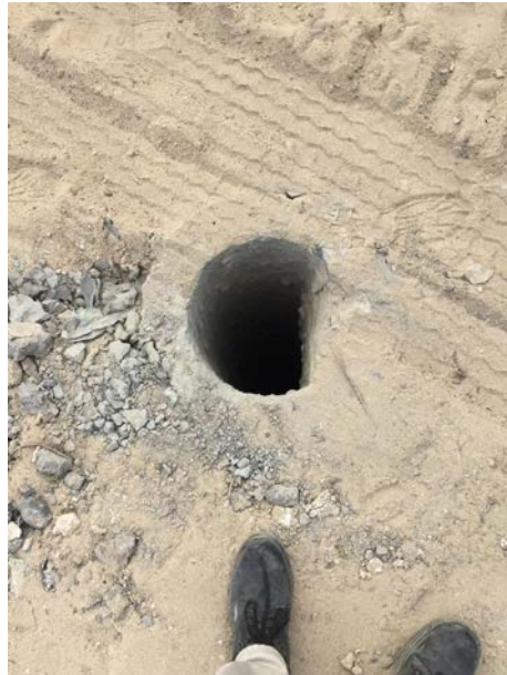
Gambar 3.9 Lubang Spun Pile
