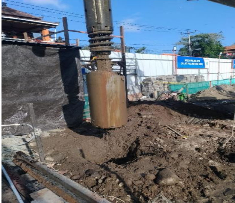
Gambar 52 Cleaning Bentonite Pile (Sumber Foto Lapangan)
