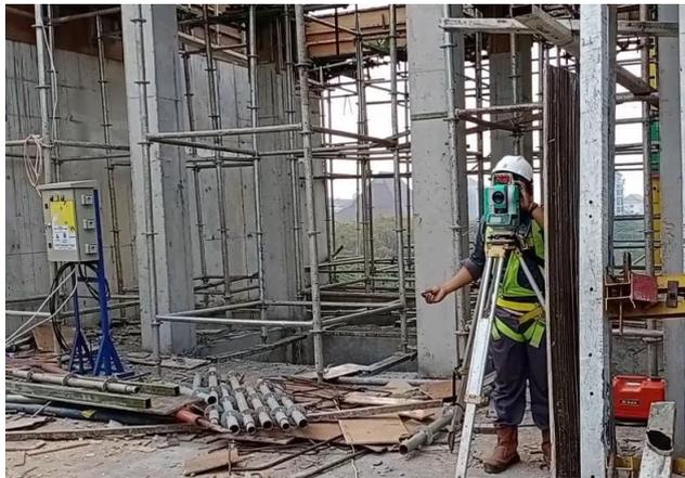
**Gambar 5. 42 Pengukuran Elevasi Bekisting**
