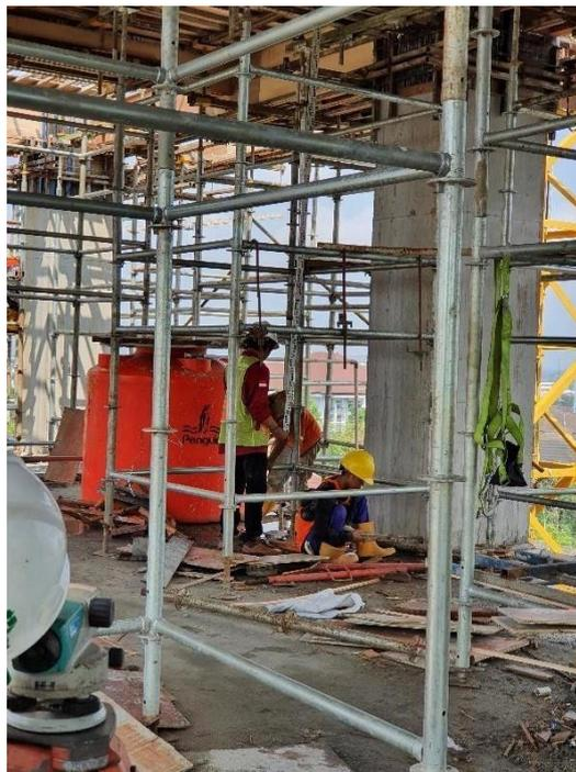
**Gambar 5. 18 Mengecek Elevasi Bekisting Pelat Lantai**
