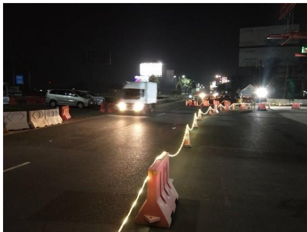
Gambar 3.9 Pemasangan Pengaman Berupa Moveable Plastic Barrier (MCB) dan LED
