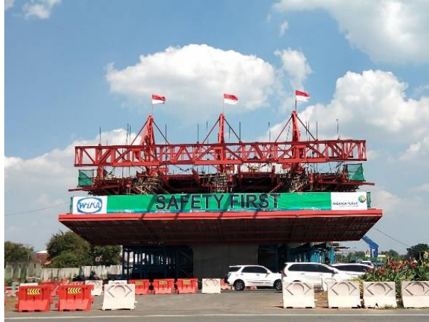
Gambar 3.36 Tampak Depan Form Traveller Segmen 1
