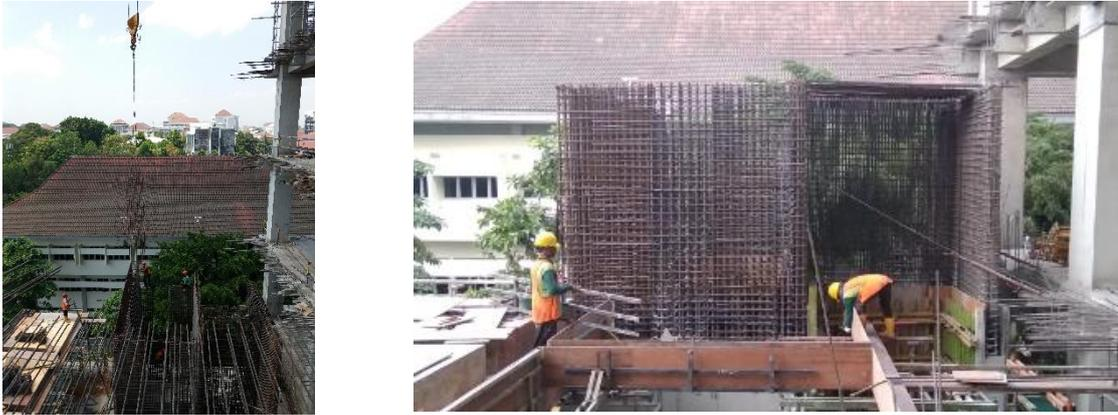
Gambar 3.21 Pekerjaan oembesian shear wall
