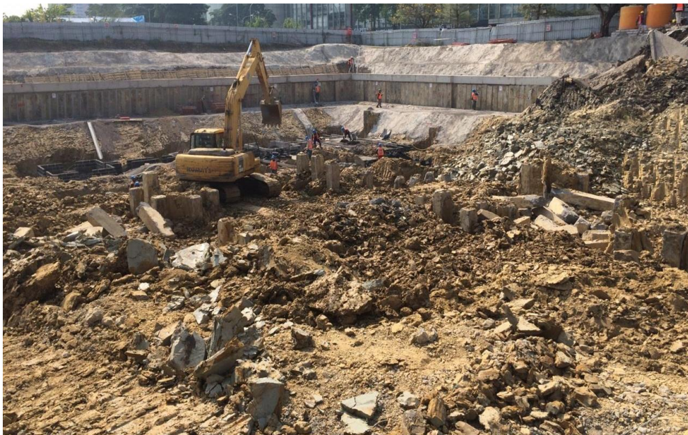
Gambar 3.12 Pekerjaan galian area tower
