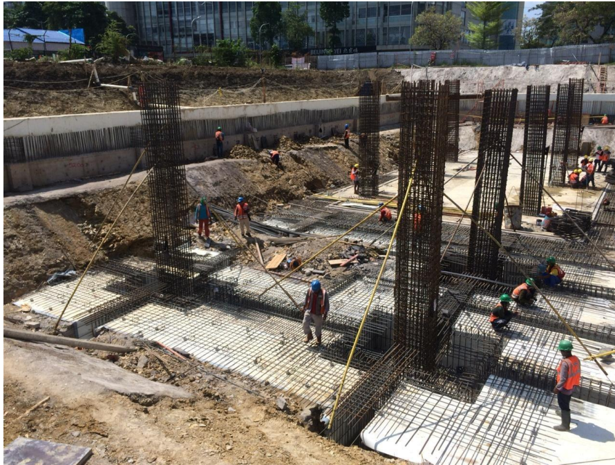
Gambar 3.16 Proses penulangan tie beam
