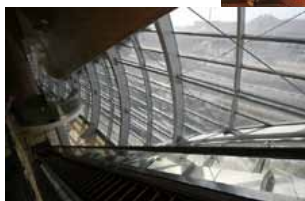
Dubai Metro, UAE Image taken by Jovana Obradovic/ITP Images
