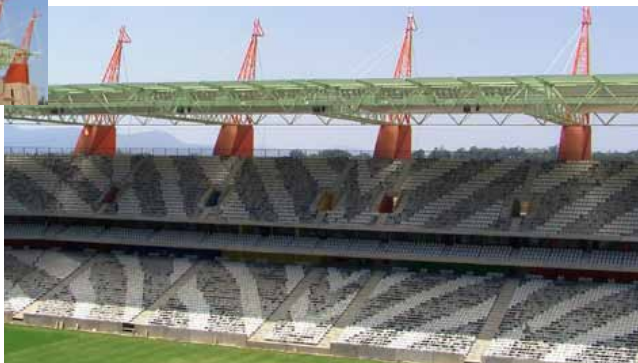
Mbombela Stadium, Nelspruit, South Africa Client - Mbombela Local Municipality Structural Engineer - Mott MacDonald
