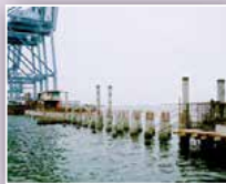
Piles for Marine Structure
