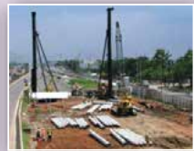
Piles Foundation for Bridges
