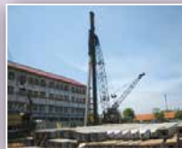
Piles Foundation for Building
