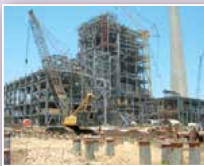
Piles foundation for Power Plant or Industrial Factory
