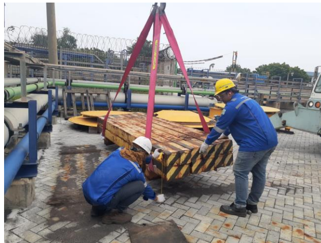
Gambar 3.14 Load Test Mobil Crane
