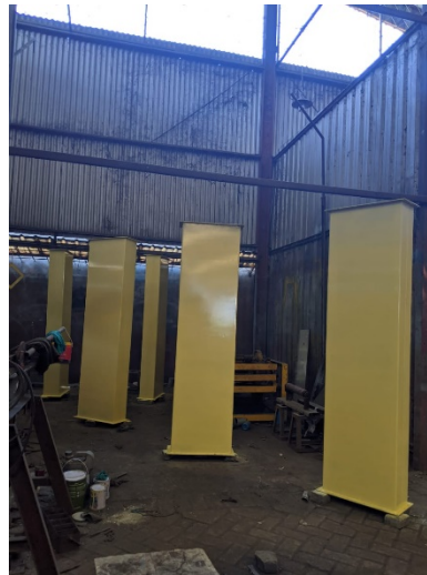
Gambar 33. Proses Pengecatan Finishing Body Bucket Elevator
