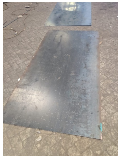
Gambar 25. Proses Pemotongan ( Cutting ) Plat Body Bucket Elevator
