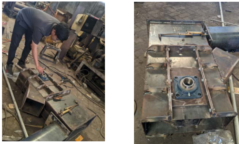
Gambar 31. Proses Sub-Assembly Bagian Tail Bucket Elevator
