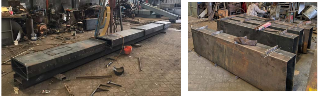
Gambar 30. Proses Sub-Assembly Bagian Body Bucket Elevator
