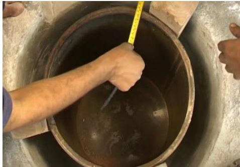
Gambar 3.5 Pemasangan Lining Former .
