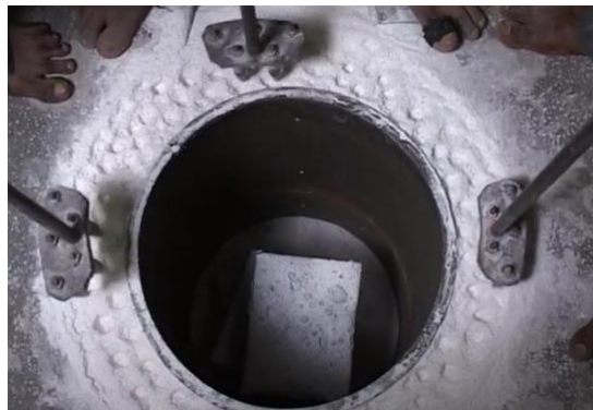
Gambar 3.6 Pemasangan Dinding Luar Lining Former .
