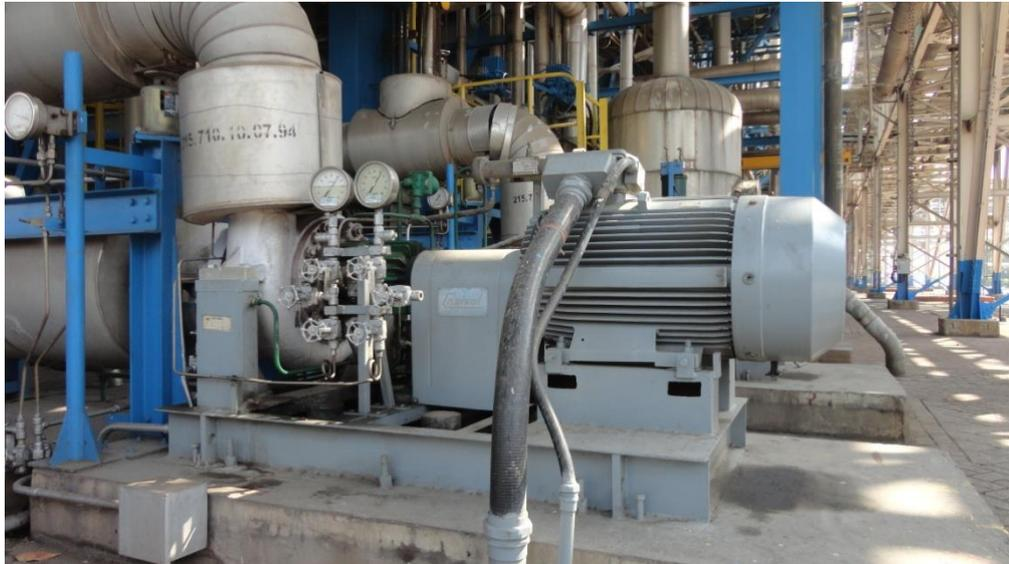
Gambar 3.9. HP Boiler Circulating Pump (BCP)
