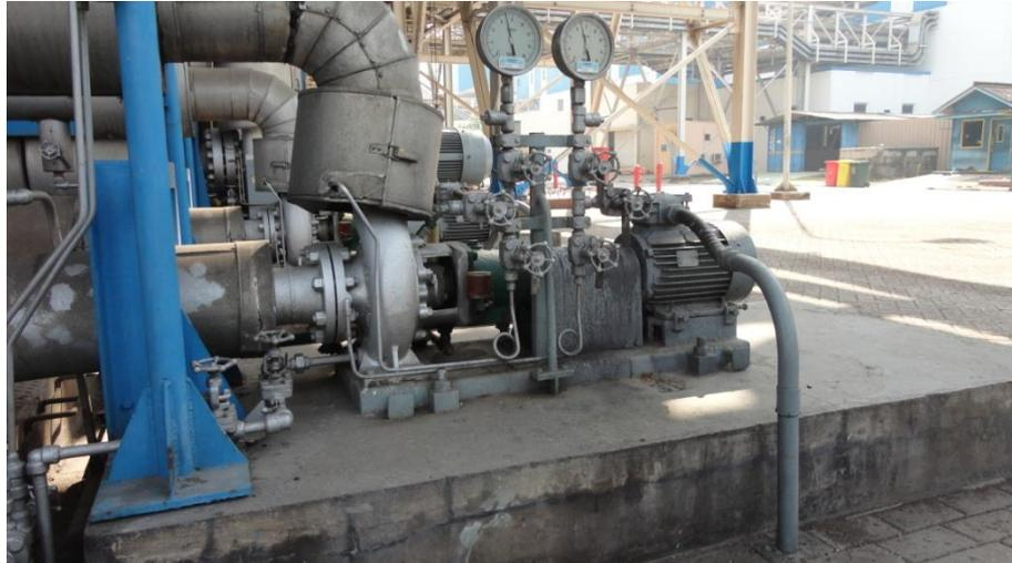
Gambar 3.11. LP Boiler circulating Pump (BCP)
