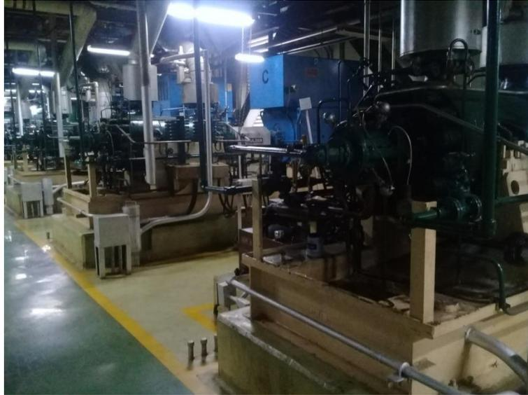
Gambar 3.15 Boiler Feed Pump
