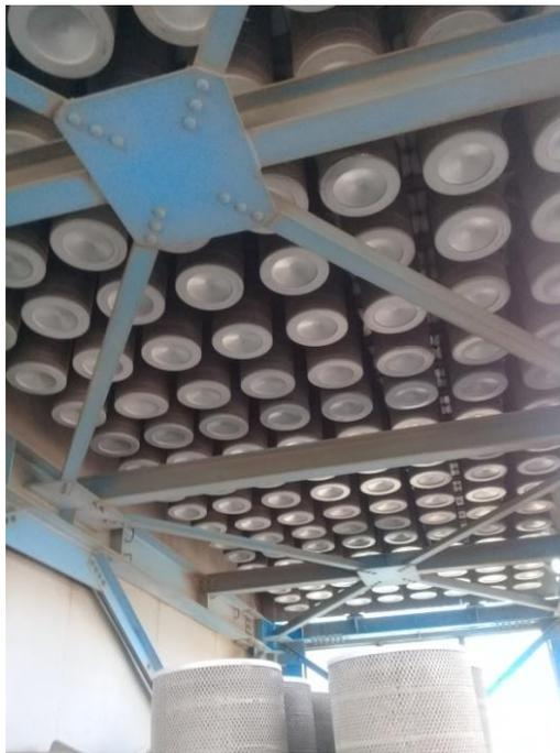
Gambar 3.3. *Intake Air Filter*
