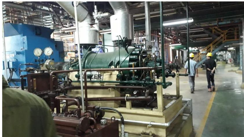
*Gambar 2 HP Boiler Feed Pump*
