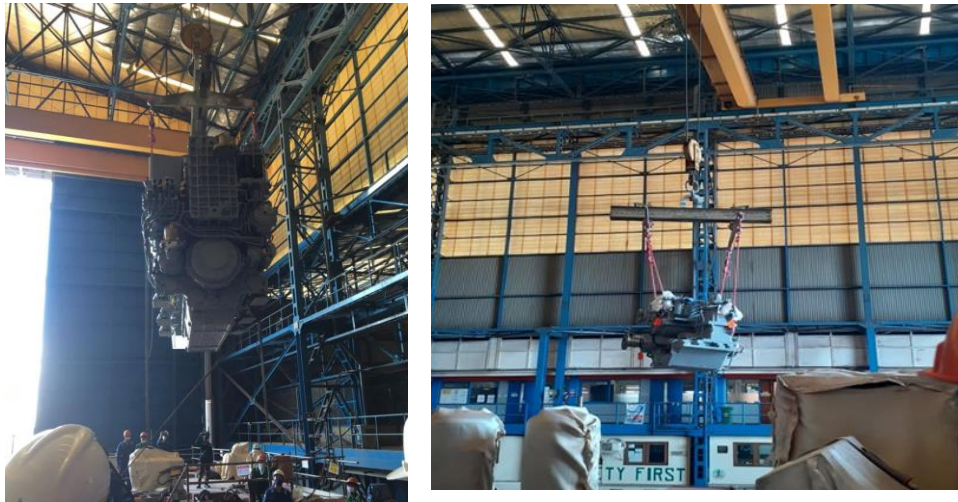
Gambar 2.13 Proses Loading Main Engine dan Gearbox
