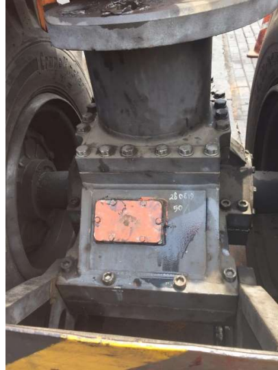
Gambar 2.21 Gantry gear travelling RTG
