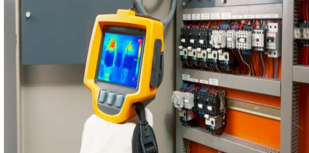
Gambar 2.59 Thermography test (Sumber:
