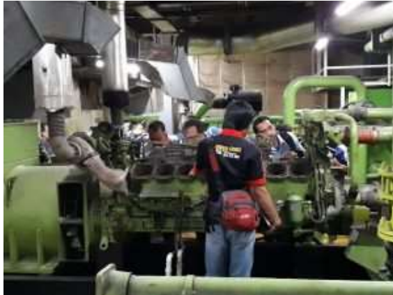
Gambar 2.65 Overhaul Generator Set
