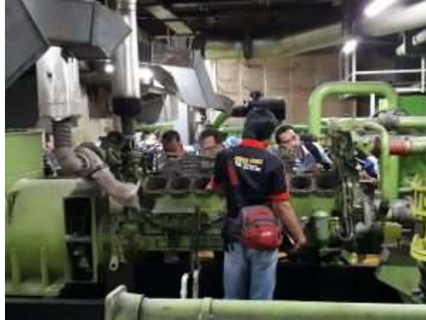
Gambar 2.65 Overhaul Generator Set
