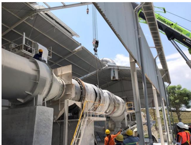
Gambar 3. 40 Proses Overhaul Rotary Dryer
