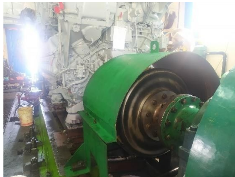
Pemasangan cover coupling
